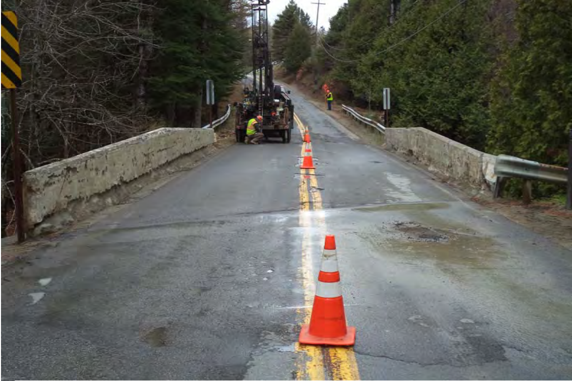
View west across the bridge
