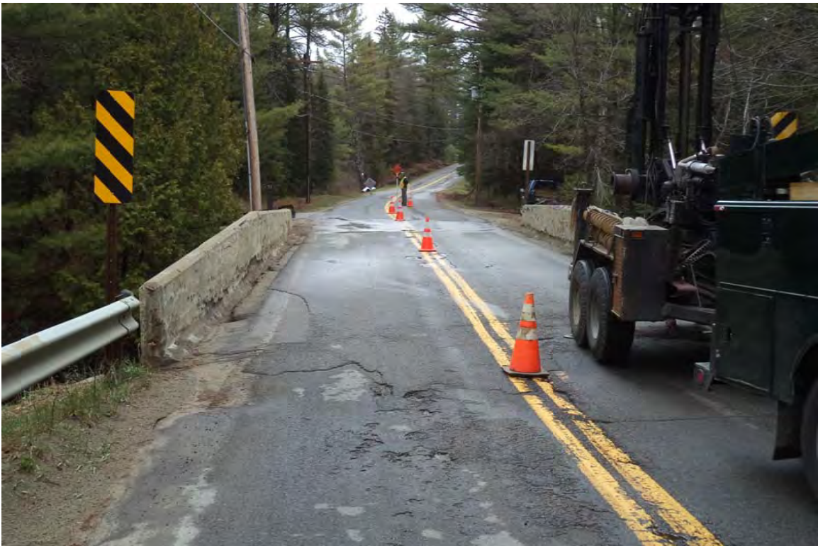
View east across the bridge
